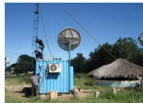
✘ Setting up containized LinkNet Resource Container in rural Chilongo, Zambia. Source: Gertjan van Stam, Macha Works ( http://www.machaworks.org/en/ )
